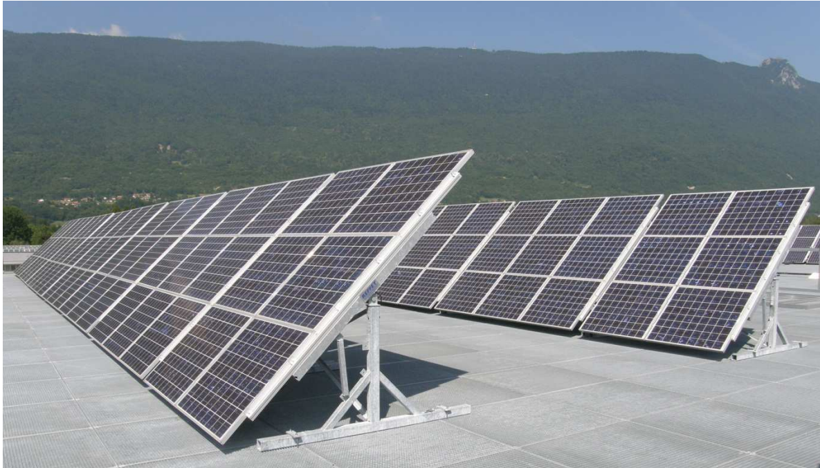
Figure 5 : PV plant 10kW peak power for green Data Net Project for PV tool forecasting tool implementation in INES
